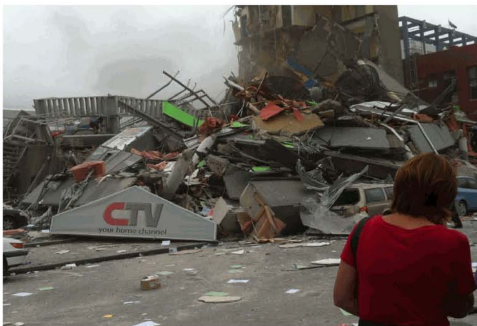
Figure 1 - The CTV Building seen from the corner of Cashel and Madras Streets immediately after the collapse, and prior to debris being shifted and removed. The escape stair on the collapsed South Wall can be seen laying on top of the rubble. Fractured Line F columns and precast concrete Spandrel Panels have fallen onto cars parked in Madras Street. A portion of floor slab from in front of the lift doors at Level 5 hangs precariously from the North Core in the distance (MSN).
