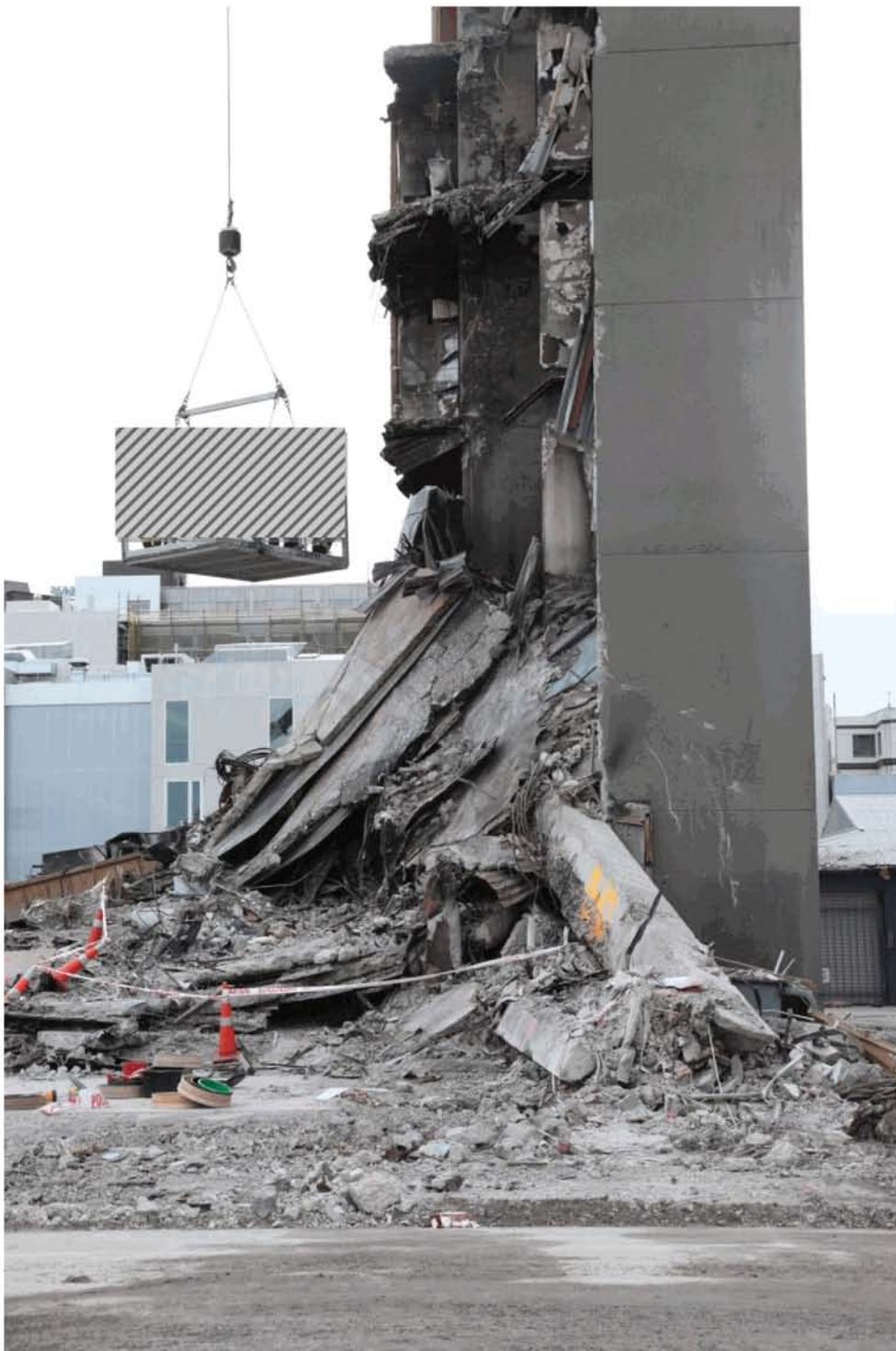
Figure 34 - North Core with Level 4 and 3 slabs laying diagonally against it.
