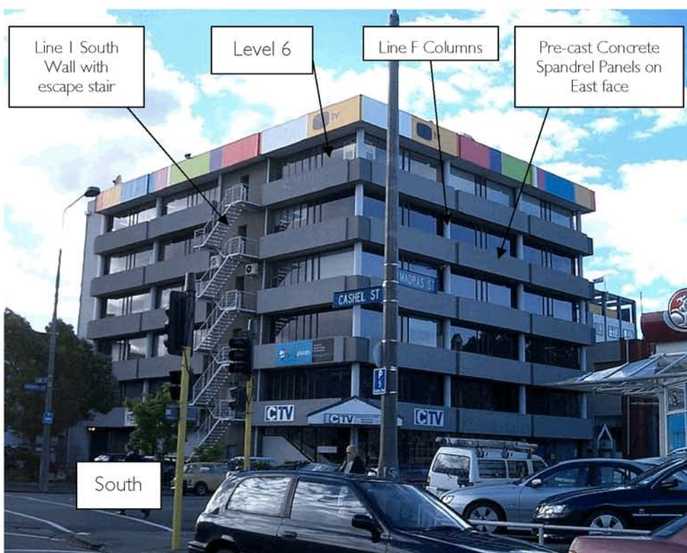
Figure 2 - Canterbury Television Building in 2004 (Photo credits: Phillip Pearson, derivative work: Schwede66) This shows some of the critical features relevant to the collapse such as the Line F columns, the pre-cast concrete Spandrel Panels, and the South Wall.
