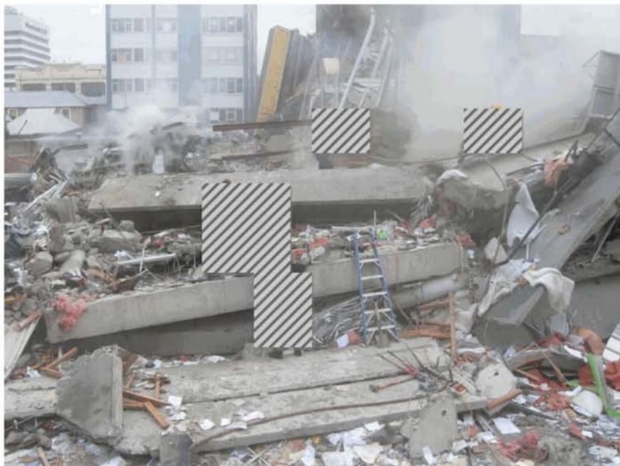
Figure 35 - Concrete Spandrel Panels, perimeter beams and columns on Cashel Street face (Line 1 / B-D).
