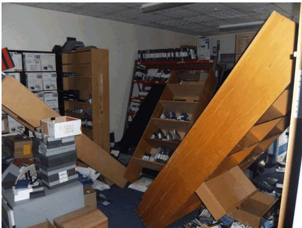
Figure 27 - Damage to office furniture on Level 2 after the 4 September 2010 Earthquake.
