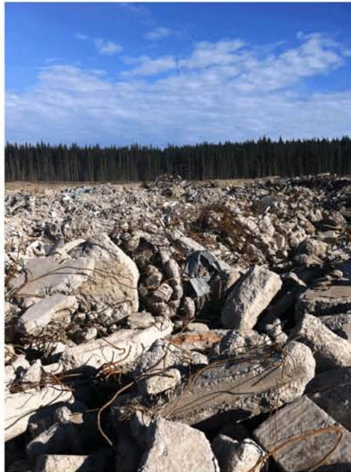
Figure 45 - A portion of the CTV Building debris field at the Burwood Eco Landfill from which columns were extracted for examination and testing.
