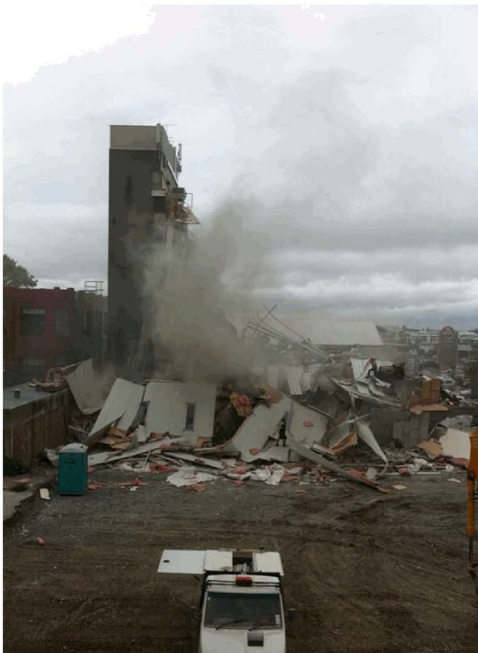
Figure 30 - View of the entire west wall on Line A from Les Mills immediately after collapse before debris removal commenced. No signs of liquefaction can be seen on the adjacent vacant site. Smoke from the fire can be seen beginning to rise. Some of the upper light weight external panels between Levels 4 and 6 have fallen northwards, possibly as a consequence of the South Wall falling north towards them. Large diagonal cracks can be seen in the Level 2 to 3 masonry infill wall at the right hand end that has fallen onto the vacant site. Roof steelwork can be seen in mid-picture.
