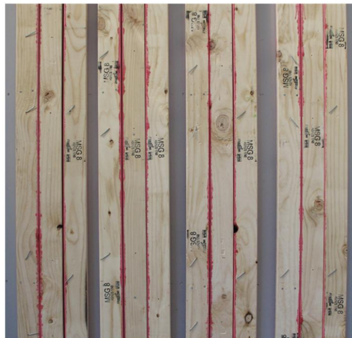
Figure 6 – The concealed faces of ‘double coat brush-on’ boron treated studs (after dismantling), unit BB1 on the left through to unit BB4 on the right. Preservative had only spread a few mm between studs from the edges that it was brushed on to.
