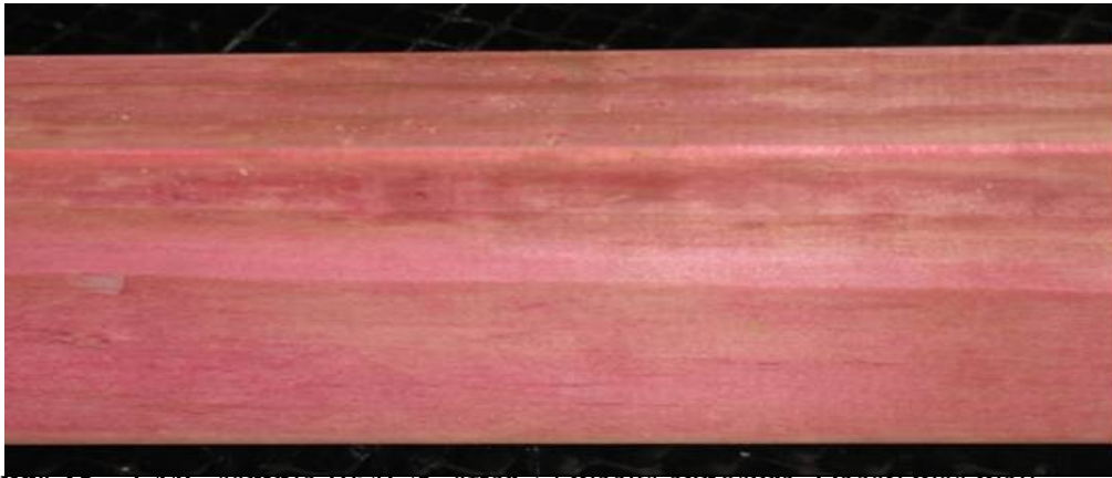
Figure 15 – LMC sample B64L/5, after 52 weeks exposure. Decay was well established on the upper edge before treatment but had not increased since.
