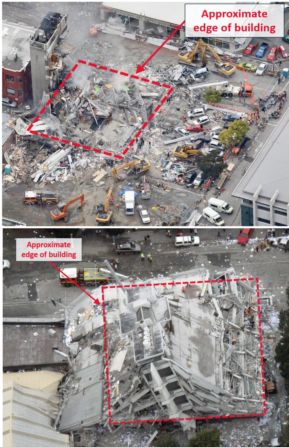
Figure 16: Aerial views of CTV and PGC buildings after collapse in 2011 Christchurch Earthquake indicating collapse debris extending beyond the building footprint.
