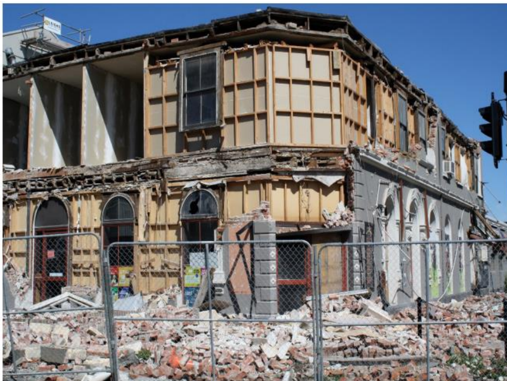
Figure 4: Collapse of the façade of a two-storey building in Christchurch, February 2011
