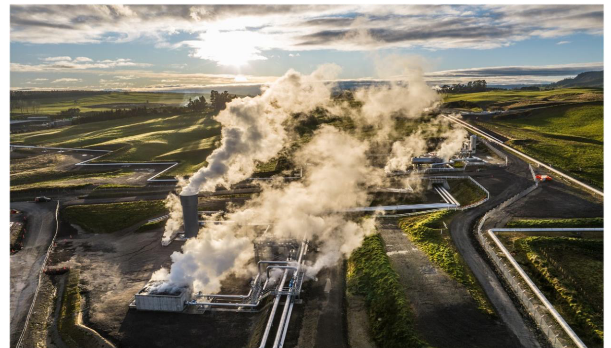
Figure 4: The Te Huka power station steaming ahead, currently piloting the reinjection of non-condensable gases (primarily CO 2 ) back into the geothermal reservoir (image supplied by Contact Energy)
