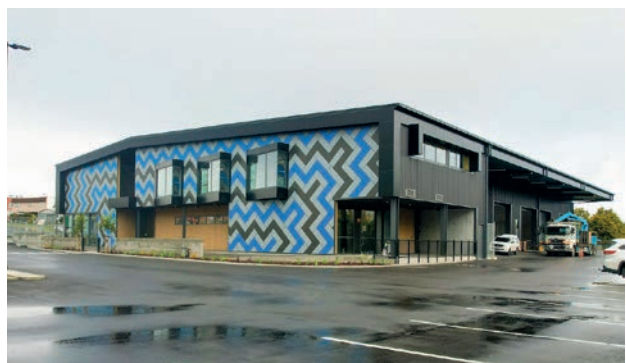
South Waikato Training Centre Complete - Tokoroa
