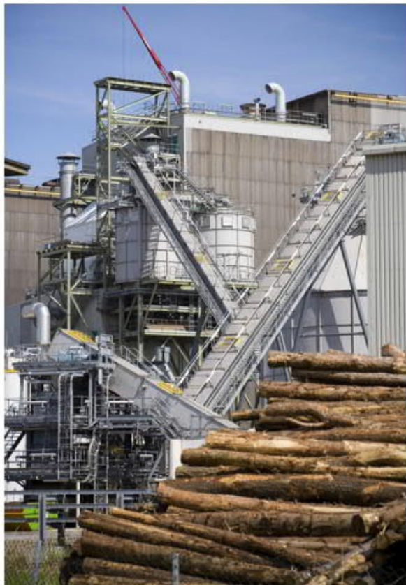
Sembcorp's Wilton 10 biomass power station in the UK. Source: Teeside Live
