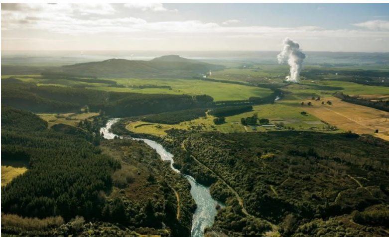
Nga Awa Purua Geothermal Station (Credit: NZ Geothermal Assn)
