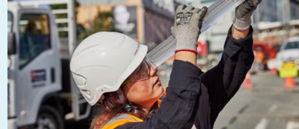
Atarangi from the City Rail Link project at Karangahape Station
