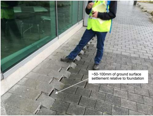
Figure 11: Ground surface settlement adjacent to the perimeter of Statistics House
