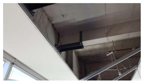
Figure 6: A typical catch bracket retrofitted in 2016
