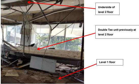
Figure 9: Fallen Double Tee unit at the first floor level
