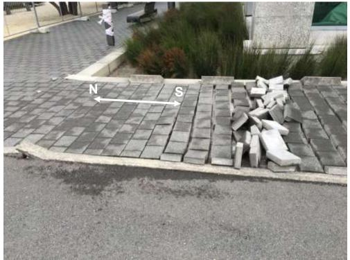
Figure 12: Compression of pavers adjacent to NW corner of Statistics House
