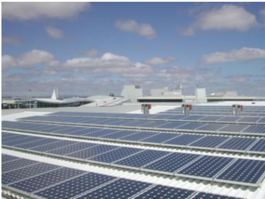
**Figure 7.1: Auckland international airport stage 1 grid tie installation, 51 kWp (Sharp modules installed by Reid Technology)**
