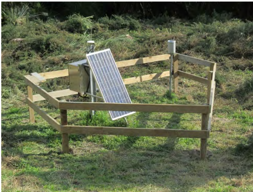
Figure 2: Example of site monitoring equipment (source: Vector Gas)
